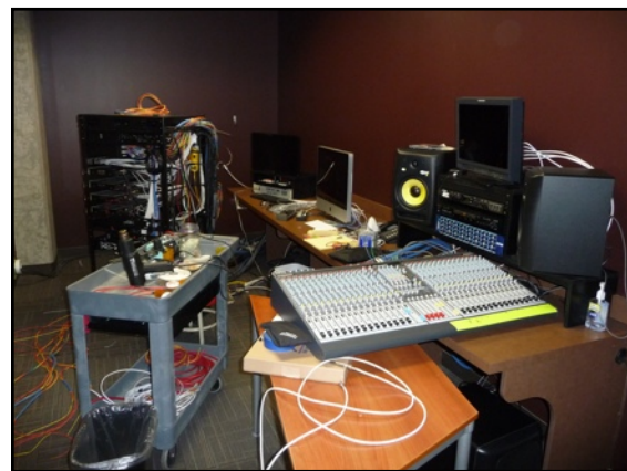
Studio Control room one--being put together!
